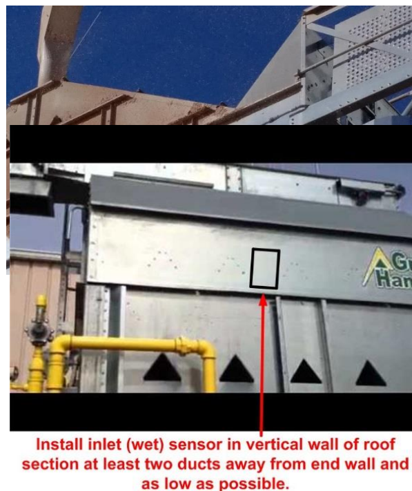
Figure 60 Sample inlet sensor installation on a Grain Handler dryer
